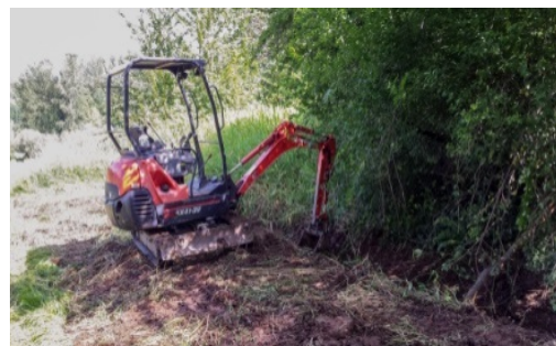
Figure 3 Mossyrock ditch cleaning
