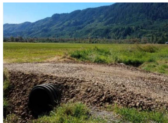
Figure 20 Davis Lake Unit culvert
