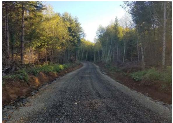
Figure 3 Peterman Mainline after reconstruction
