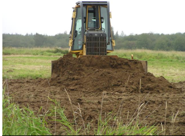
Constructing 5 th and final ditch plug – Chinook Unit
