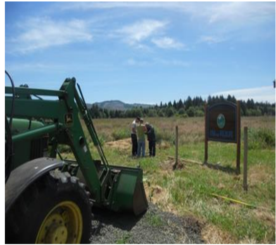
Kiosk and Access Construction 2015
