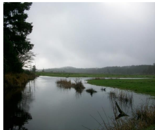
Main control structure flooding ditched John's River
