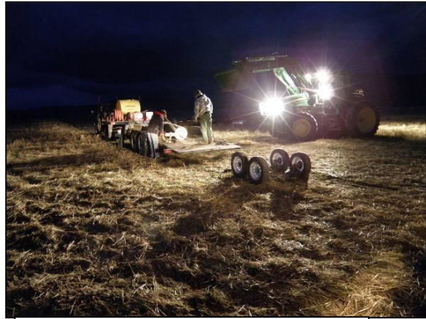
Unloading equipment for grass seeding, November, 2010.
