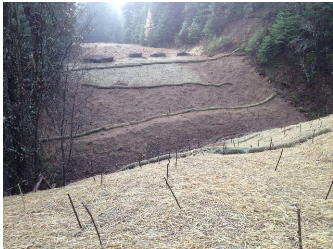
Location where an undersized culvert was removed.
