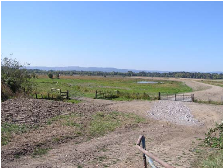
A levee was completed to reestablish 120 acres of wetland habitat
