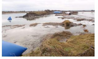
inside the dike to keep the island from flooding once the dike failed. The coffer dams protected the site until the weekend of Easter 2010 when one of the coffer dams failed allowing tidal flooding.
