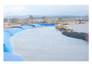
WDFW was concerned about the failing dike system and the likelihood that the winter storm tides would further degrade the dike system. In an effort to protect the site for potential project implementation during the 2010 construction season, temporary coffer dams were installed just
