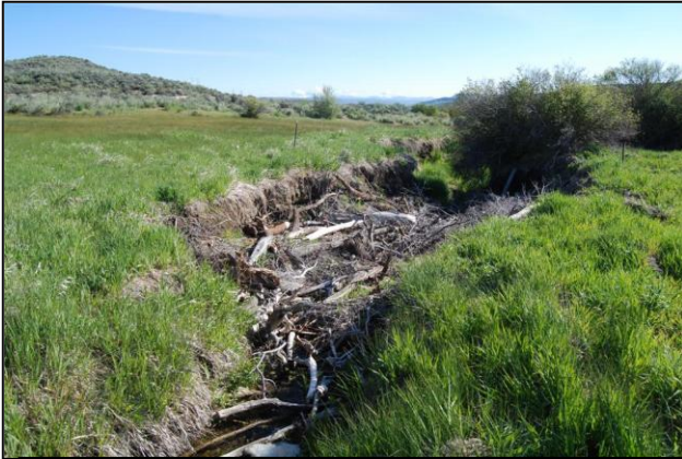
West Foster Creek Head Cut Erosion and “Brush Plug”
