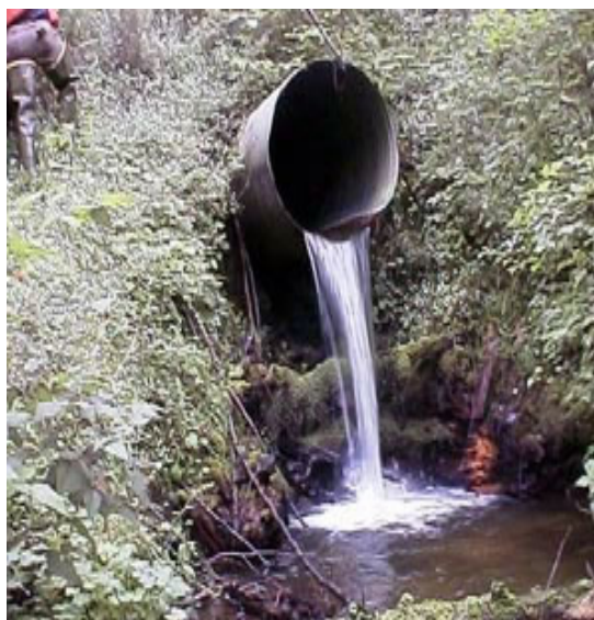
Figure 3-7. Drainage culvert projects are one type of activity contained in the HPMS database.
