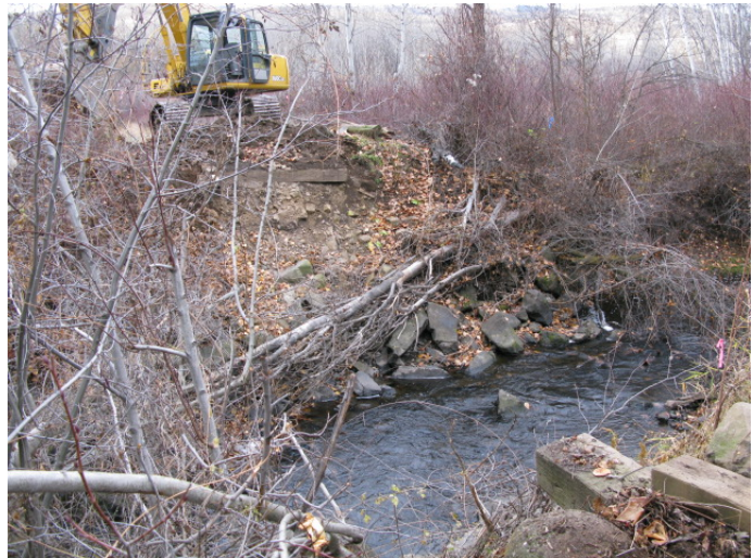
Hardy Canyon Bridge Removal
