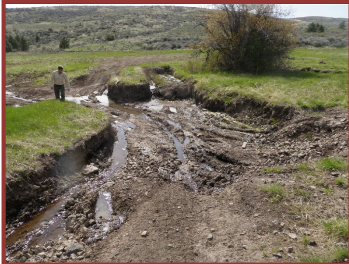
Ridge Road/Oasis Spring – Proposed for renovation to protect habitat
