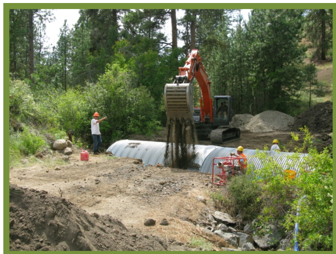
Middle Fork Culvert Replacement on Newland Road
