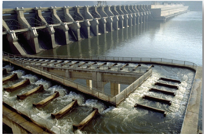
Fish ladder at John Day dam. USACE photo
