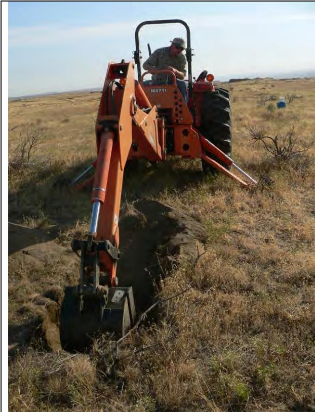
Backhoe digging main hole for burrow chamber; the bottom of the burrow chamber will be 36 inches below ground level.
