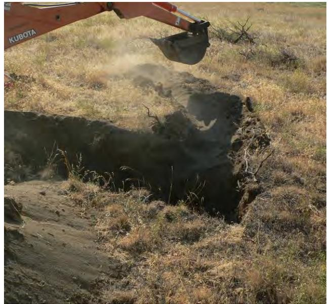
Trench for the burrow tunnel is done with a sweeping motion of the backhoe bucket. In this image it is a left-swinging and upward motion. This gives the trench an appropriate arc for the main tunnel. Some hand digging may be necessary (to get the trench deep enough) right where the main tunnel meets the collar/burrow chamber.
