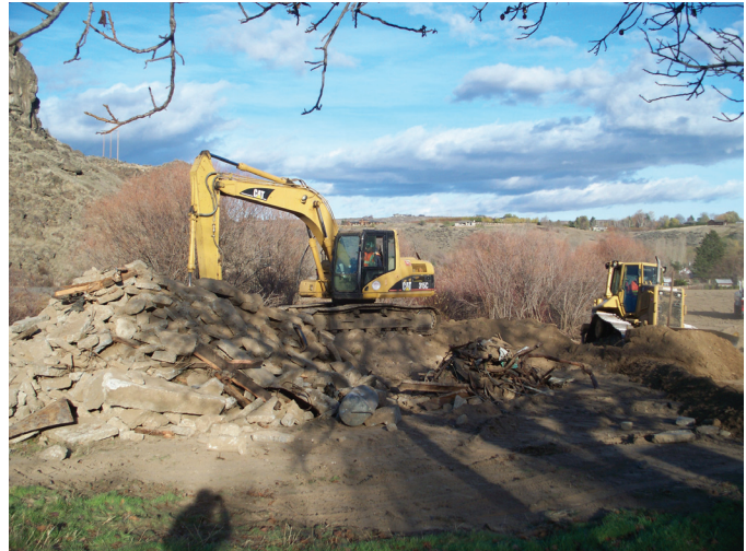
A contractor removes concrete and debris from Cowiche Creek, 2010.
