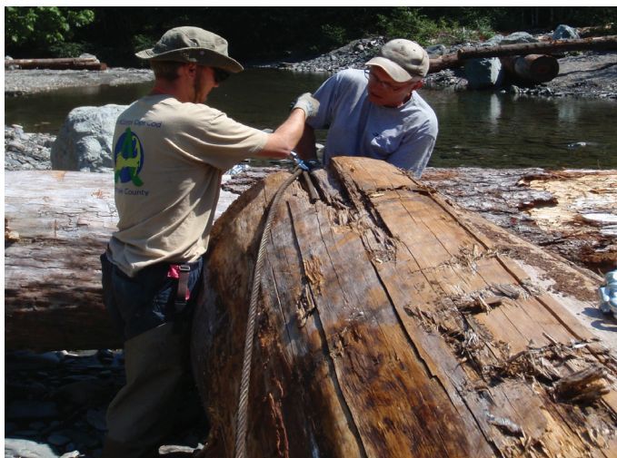
SFEG staff secures cables to re-create log jams in Finney Creek
