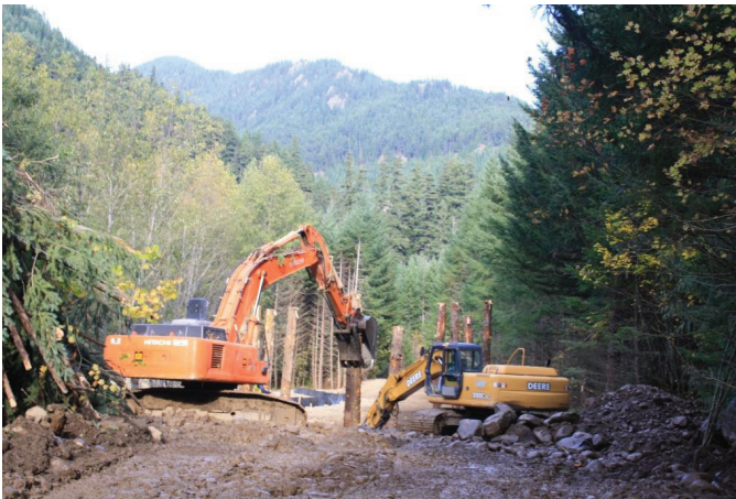
Driving piles at Greenwater River
