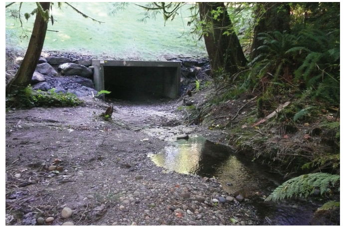
Jarrel Cove post construction
