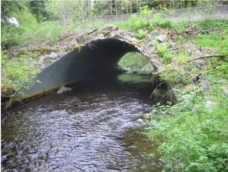
Figure 2.1: No-slope culvert, Johnson Ck, Mosquito Lake Rd.
