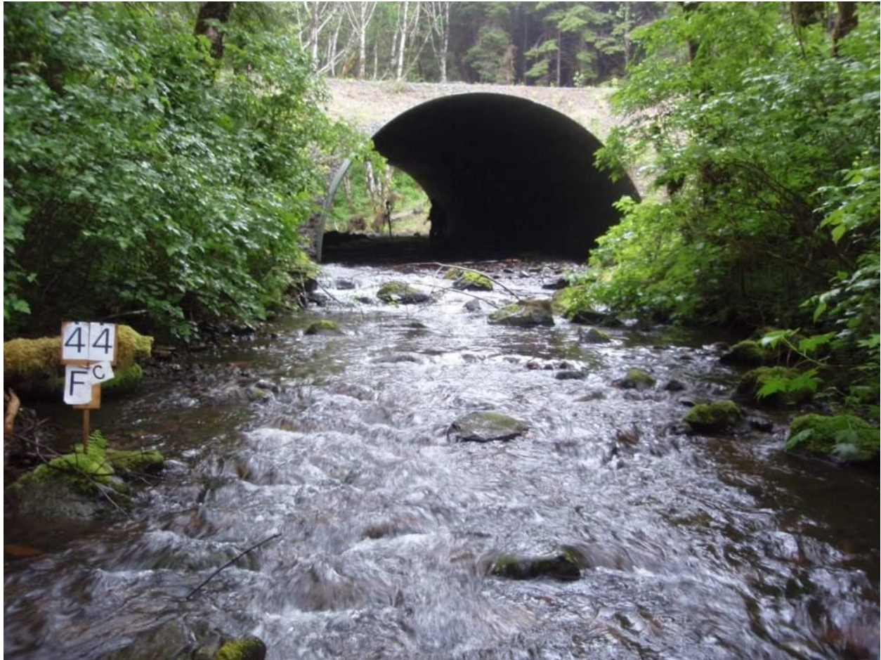
Figure 3.1: Stream simulation culvert, Newberry Ck.
