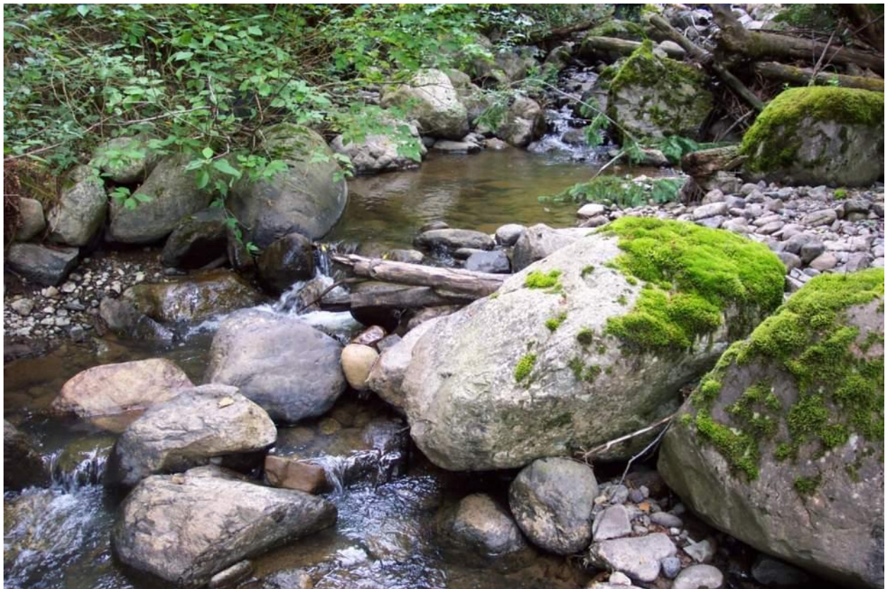
Figure 6.4: Crazy Ck roughened channel, constructed 1994.
