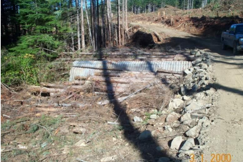
Figure 8.1: Temporary culvert. Non-merchantable logs are used as fill around the culvert to make it easier to remove and to protect the culvert. Road fill is kept to a minimum and native soils are used.
