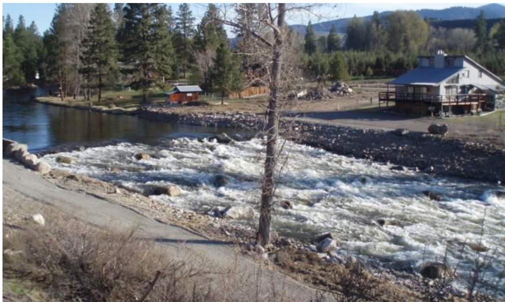
Figure 6.5: Fulton irrigation diversion with roughened channel. Irrigation intake is to the left in the photo. This type of roughened channel is often referred to as a rock ramp and its design has been described by Aadland (Bates and Aadland 2006) and Newberry (Newbury and Gadoury 1994).
