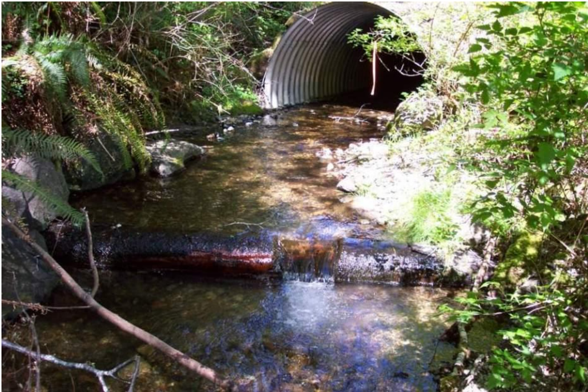
Figure 7.7: Log control used to control grade at the outlet of a culvert.
