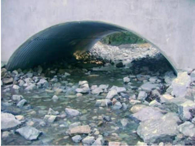
Figure 6.6: Roughened channel culvert in California, photo Michael Love and Associates. Bed is composed of angular material, which is the least preferred, and stream banks could have been reinforced with biotechnical methods rather than rock.
