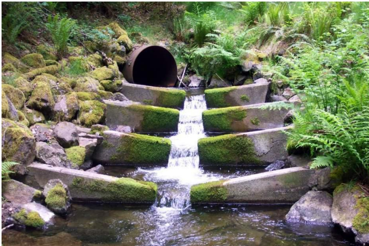
Figure 7.9 Fishway at the outlet of a baffled culvert, Dickerson Ck. This fishway is composed of precast concrete weirs formed to a pool and chute configuration.
