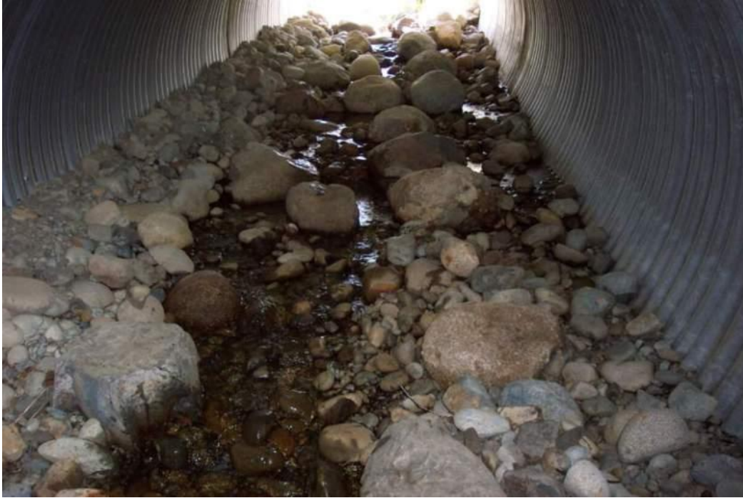
Figure 6.8: Roughened channel culvert. Shown at low flow. Bed material is rounded, but the bed should be countersunk deeper to be more robust.
