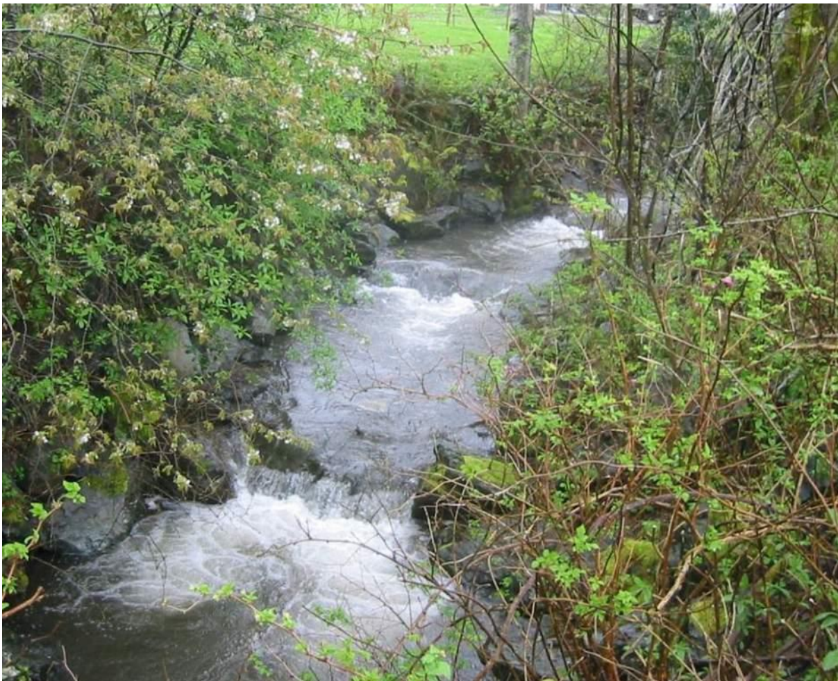
Figure 7.8: Boulder controls to maintain grade at a culvert replacement site, NP Ck. These controls are 13 years old.
