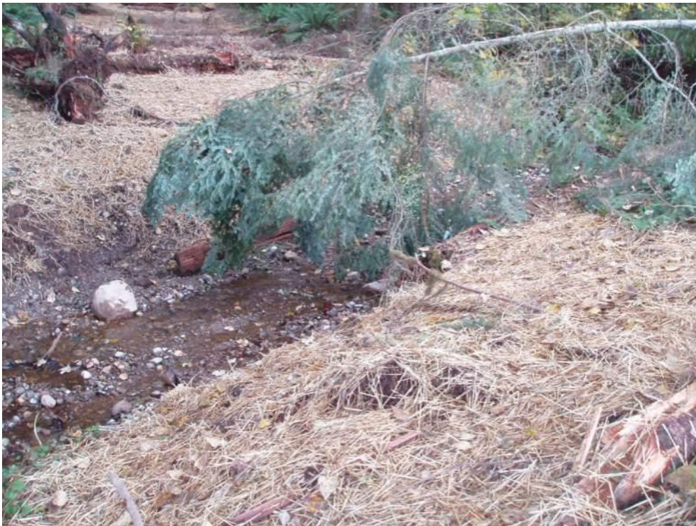
Figure 8.2: Temporary culvert site after removal. All traces of the temporary fill are removed and straw is placed on the banks to decrease erosion. Wood and slash are added to improve habitat.
