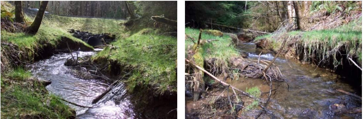
Figure 7.2: Regrade resulting from culvert replacement.
