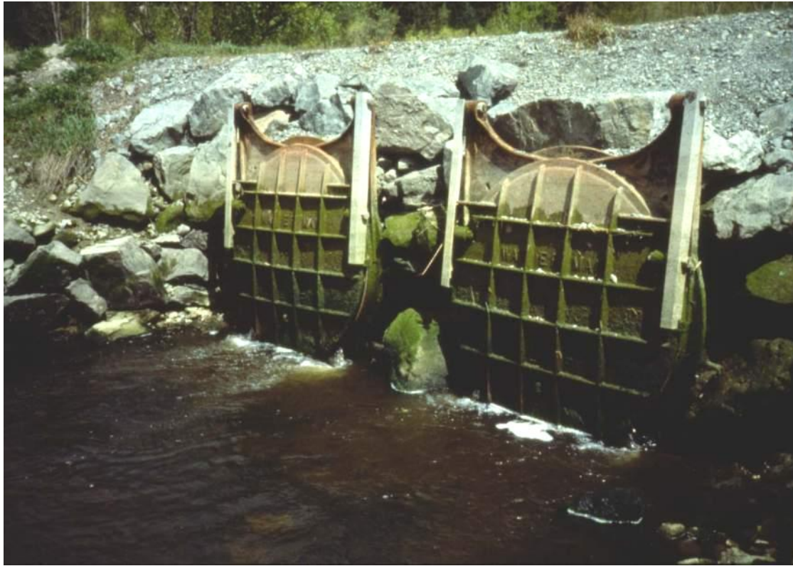
Figure 10.1: Cast iron top-hinged tide gates prevent nearly all upstream fish migration.
