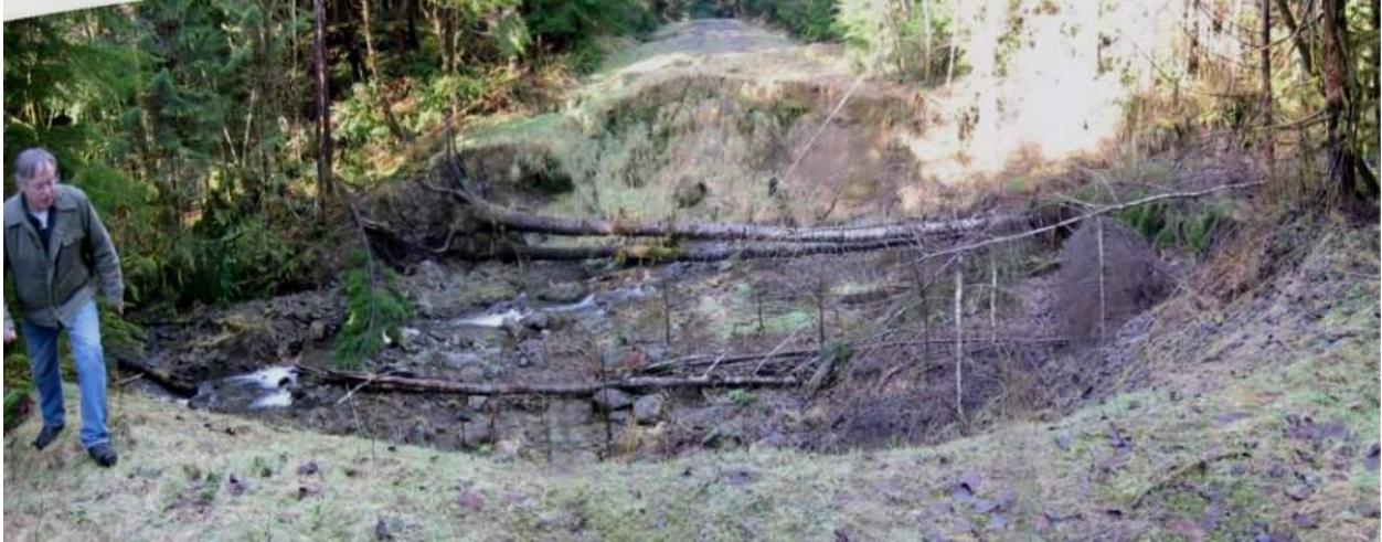
Figure 8.1: Culvert abandonment site showing full floodplain excavation and placement of large wood in excavation.
