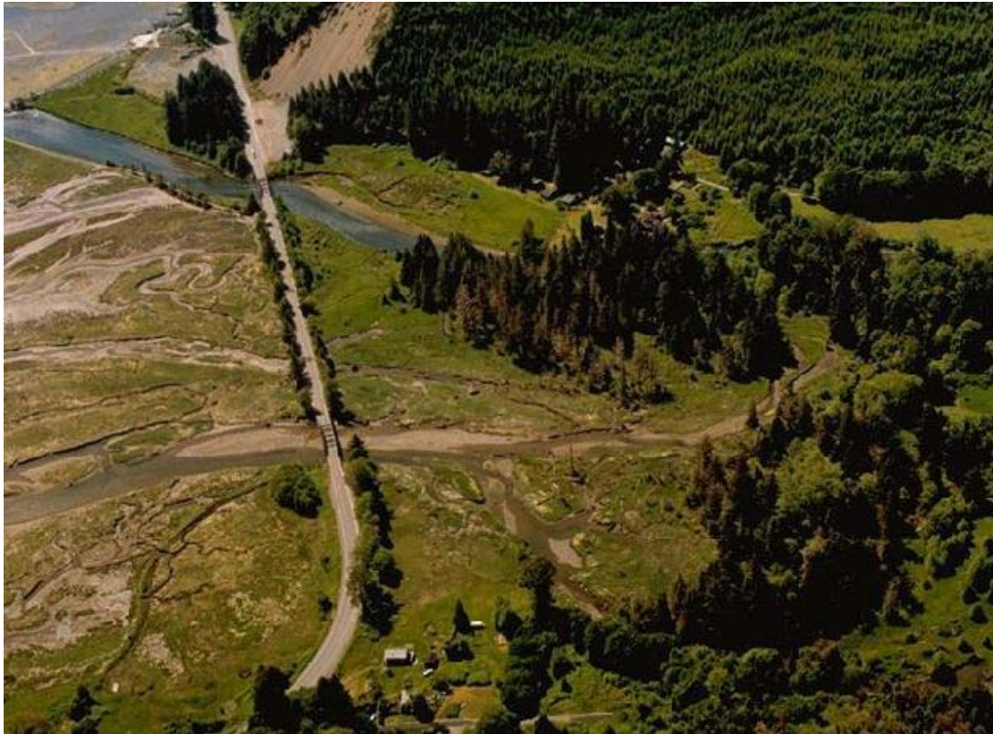
Figure D.1: US 101 crossing of the Hama Hama River delta (Washington Dept. of Ecology photo).
