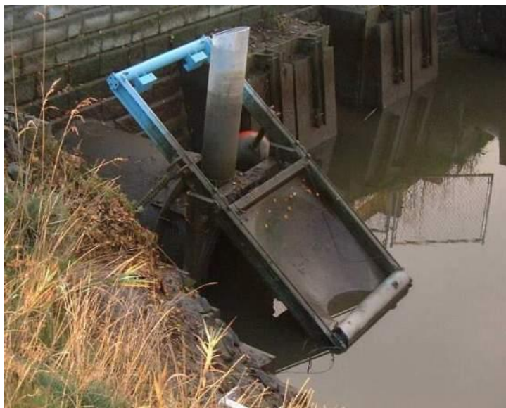
Figure 10.5: Edison Slough self-regulating tide gate.
