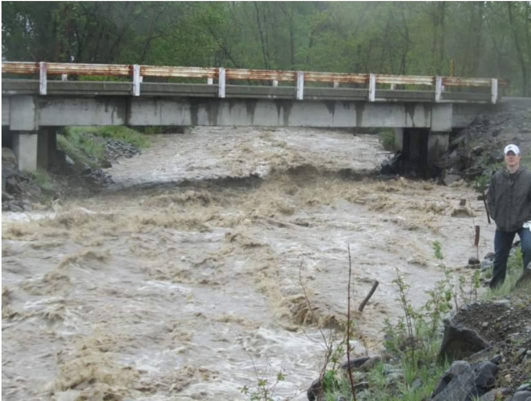
Figure 6.7: Taenum Ck. Bruton irrigation diversion. This roughened channel is shown at high flow. The design must consider flow conditions like this to ensure that the channel does not degrade. Photo Paul Tappel.
