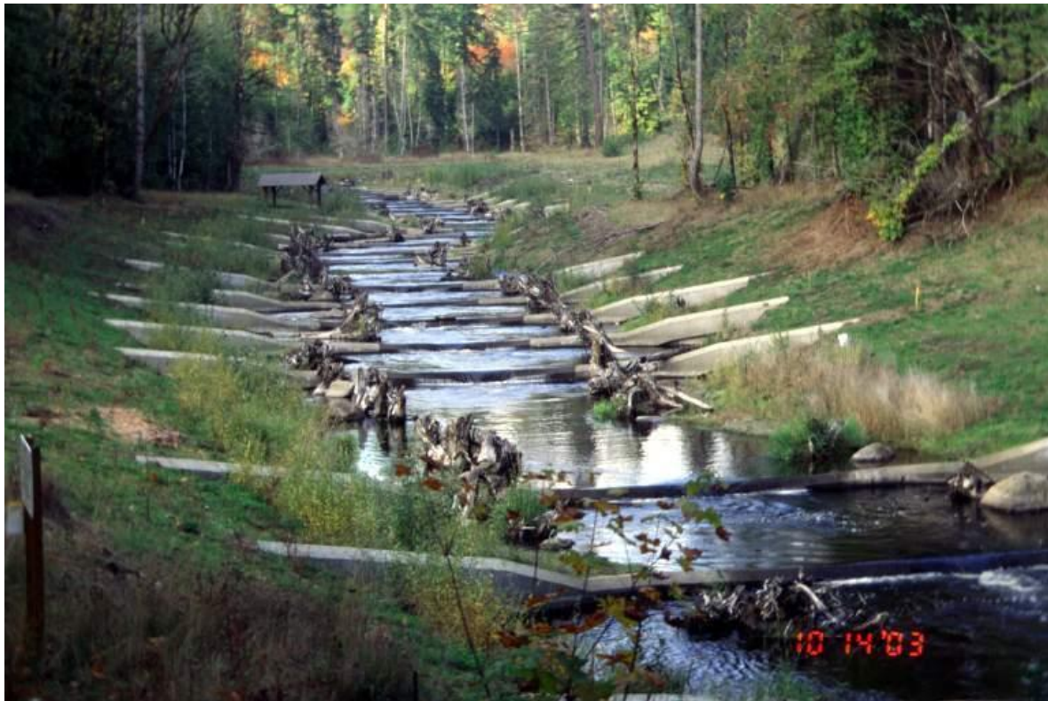
Figure 7.6: Soldier pile and cast concrete grade control structures at a dam removal site on Goldsborough Ck. This site has now become thickly vegetated and has a more stream-like appearance.
