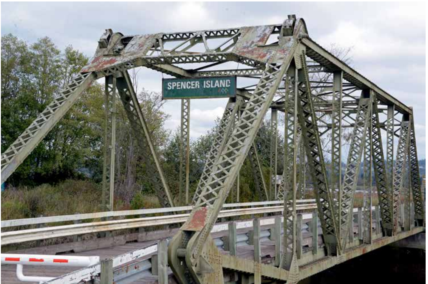
Spencer Island Bridge Photo by Alan Bauer
