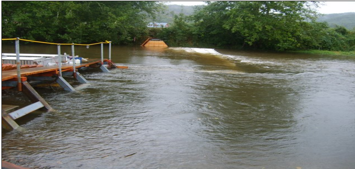
Figure 15. Photo of Grays River Weir taken on October 4, 2008 after resistance board portion of the weir had submerged (564 cfs) (data from WDOE 2008).
