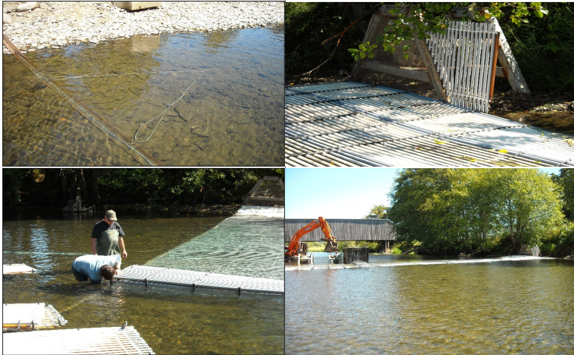
Figure 4. Photos of the installation of the Grays River Weir, 2010.
