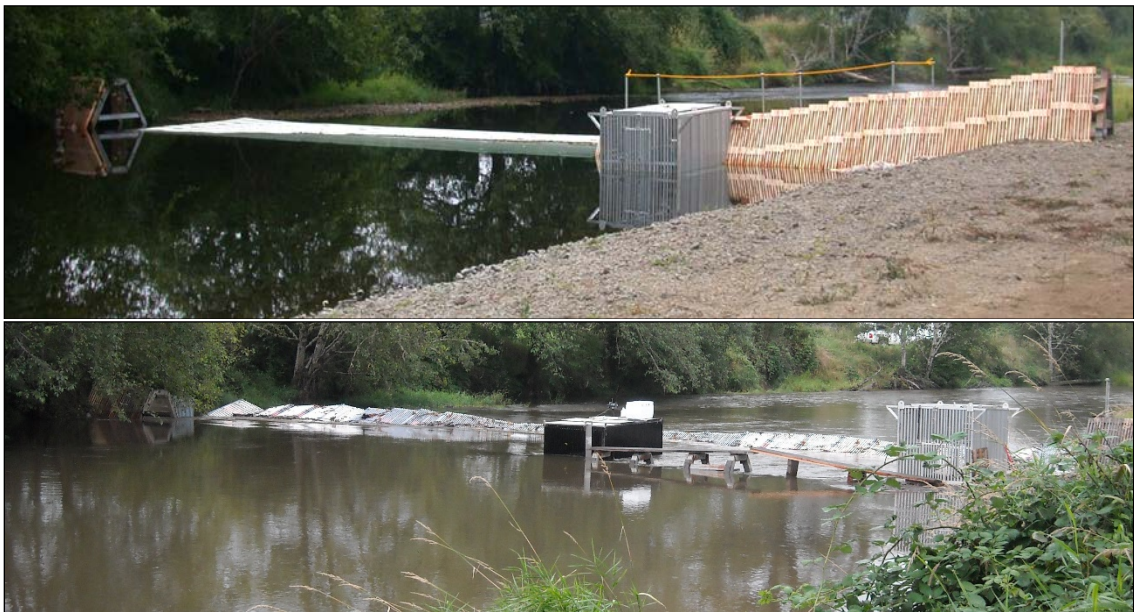
Figure 18. Photo of the Grays River Resistance Board Weir. The top photo was taken in 2008 and the bottom photo was taken in 2010.
