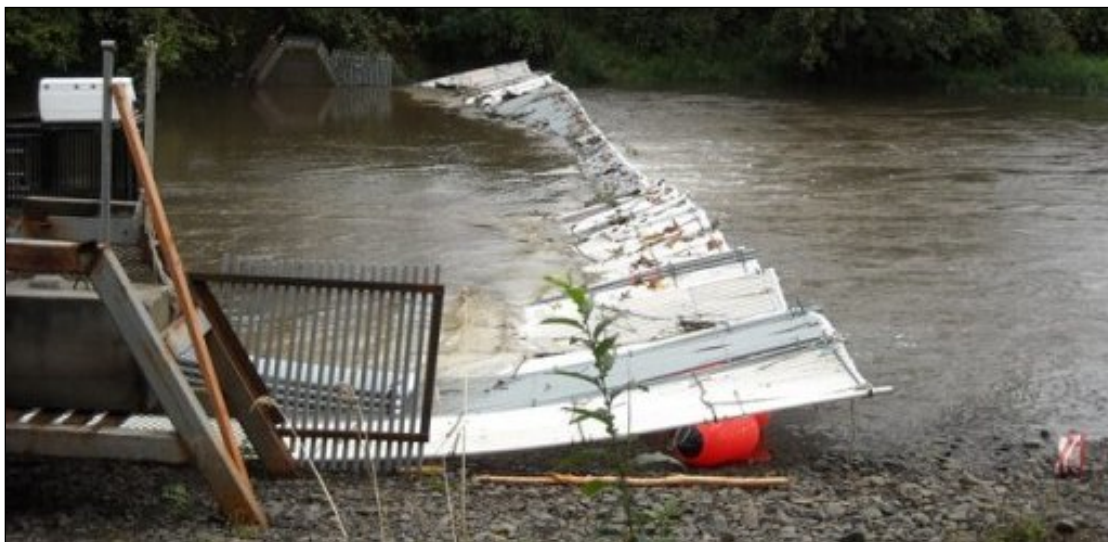
Figure 5. Photo of the Grays River Resistance Board Weir, 2010.
