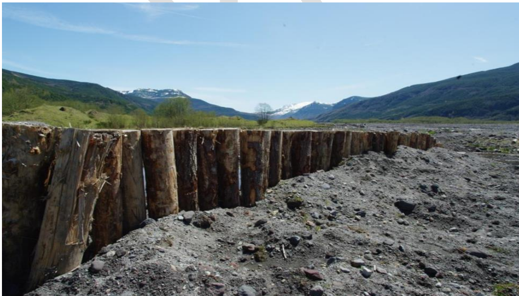
Pile dike structure. Photo by Daren Hauswald
