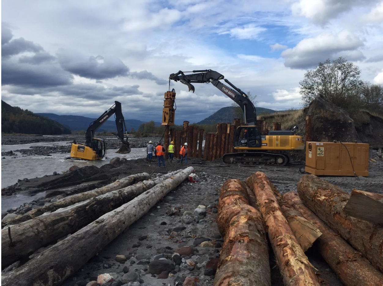
Pile Dike Construction Mudflow Unit – Photo by Daren Hauswald
