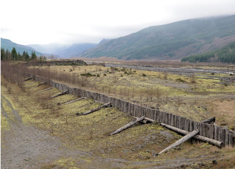
Streambank protection at Mudflow Unit. Photo by Alan L. Bauer.
