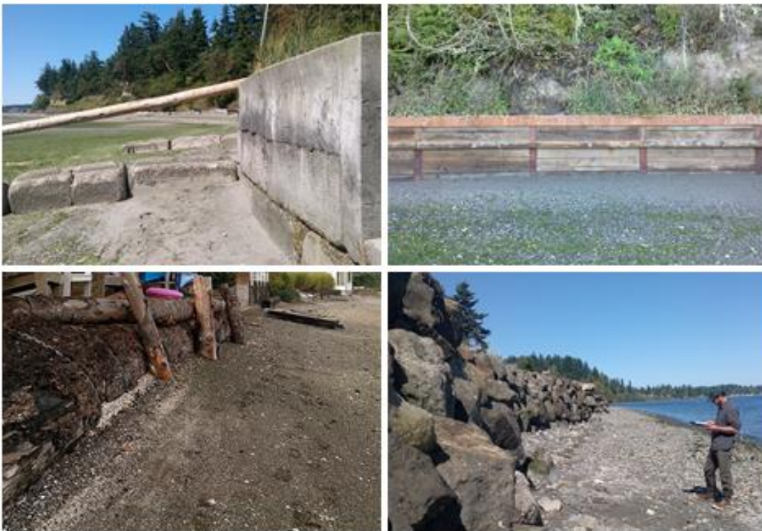
Figure 4.1. Images of various hard armor designs. Top left: concrete wall with ecology block groins; top right: vertical wood wall; bottom left: anchored log and vertical wood piles; bottom right: rock revetment
