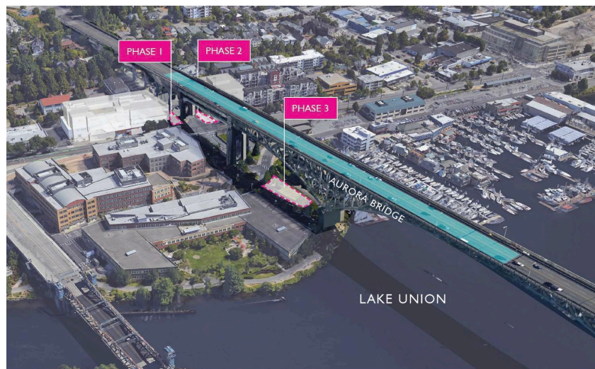
Figure 3. The swales are built adjacent to the Aurora Bridge, a historic structure in Seattle where all five of the region’s salmon species swim to reach the network of rivers and streams for spawning each year. Image credit: Weber Thompson.
