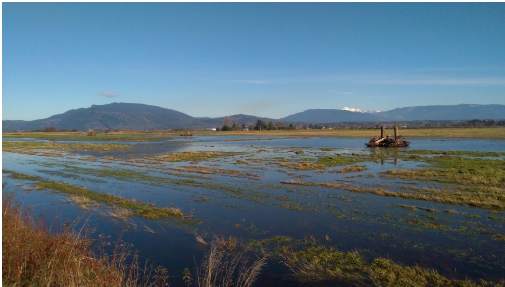
Samish River Unit restoration.
