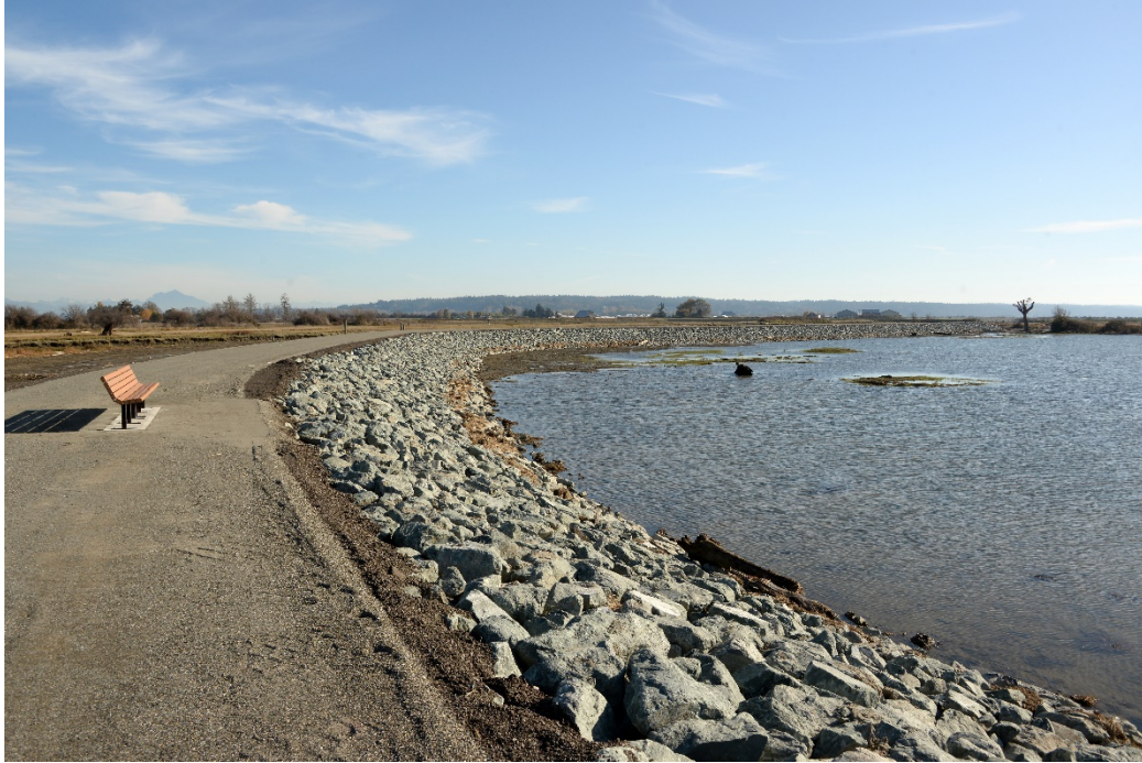
Leque Island - 2019 new dike constructed. Photo by Alan L. Bauer.
