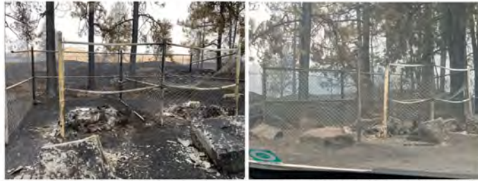
Figures 17 & 18: The toilets at West Medical Lake are hazardous since they are just open pits now. Toilet debris covers the pits and will need to be cleared and new toilets installed. The photos above show the melted fiberglass housing of four outhouses covering the inground waste tank. – Photo credit, Daniel Dziekan, Water Access Manager
