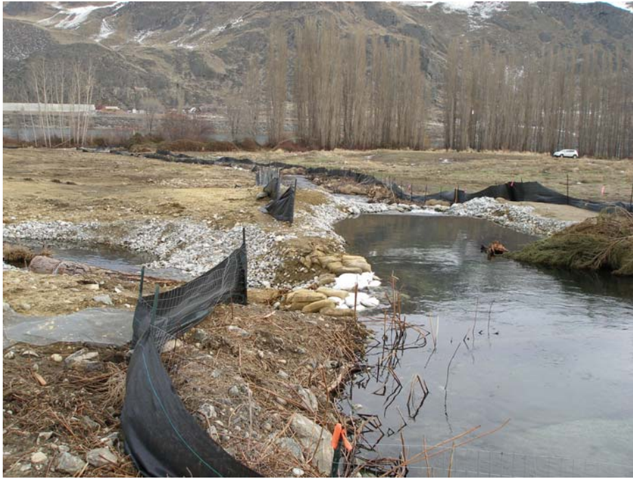
Diversion (on left) of Water from Original Channel of Beebe Creek to New Channel
