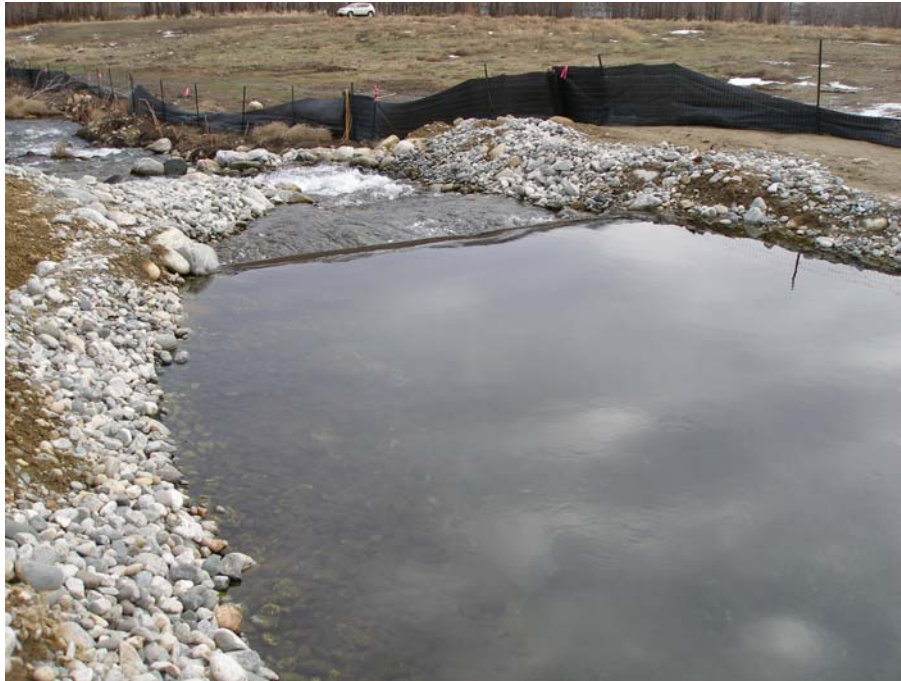
Log Weir at Backwatering Pool of Original Channel of Beebe Springs Creek below Highway 97 Culvert
