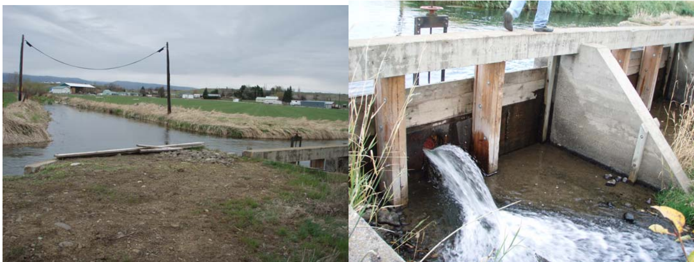
Figure 2. These photos illustrate the current conditions at the project site. Currier Creek is checked up via a concrete and wooden dam board structure, preventing fish passage and it intermingles with irrigation water in the EWC Canal.
