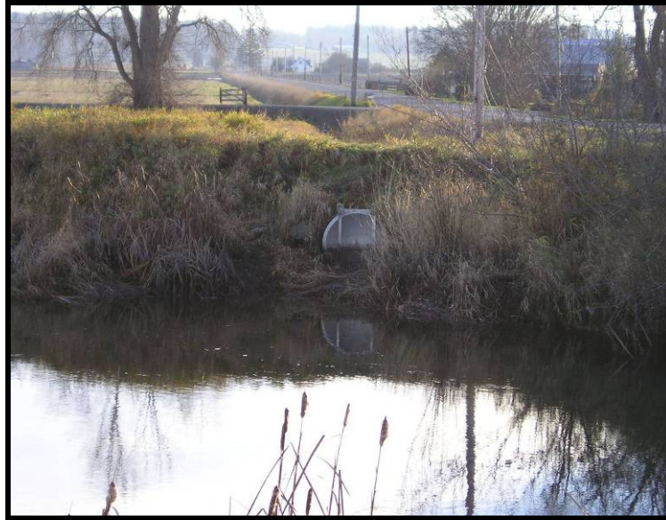
Figure 1-3. Floodgate, Drainage District 25 – Samish River system.
