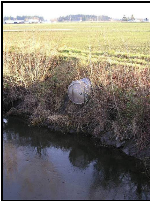
Figure 1-2. Floodgate, Drainage District 25 – Samish River system.
