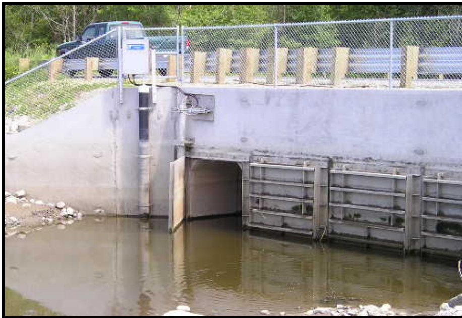
Figure 4-2. McElroy Slough Automatic Regulating Tidegate, “Aberdeen” style gate, open at a -2.7 foot tide event (County owned tidegate complex).
