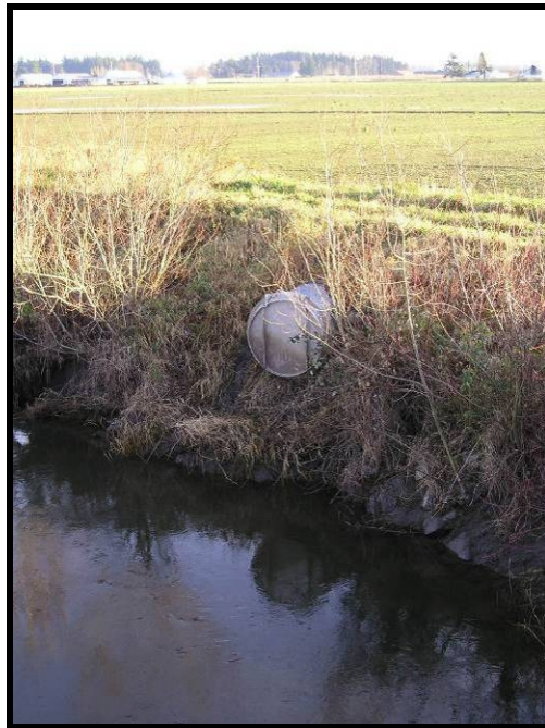
Figure 1-2. Floodgate, Drainage District 25 – Samish River system.
