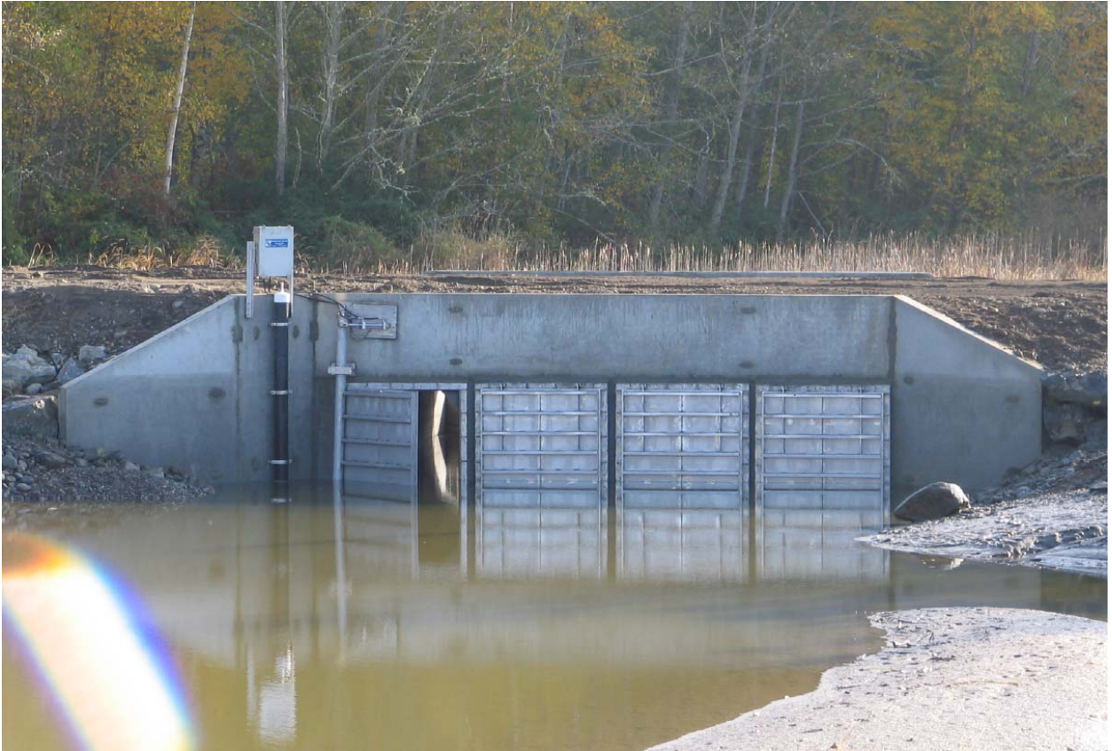
Figure 3. Recent Side-Hinge Flood Gate Installation (Golden Harvest, 2006)
