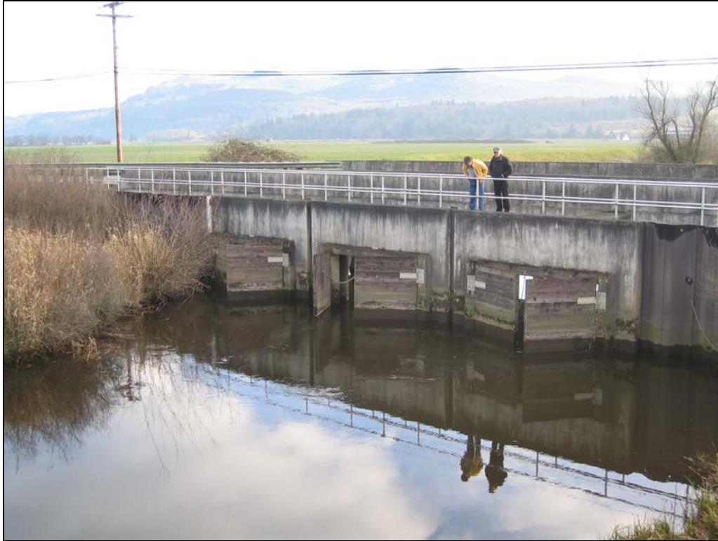
Figure 5. Existing Fisher Slough Floodgates (looking upstream from railroad bridge)
