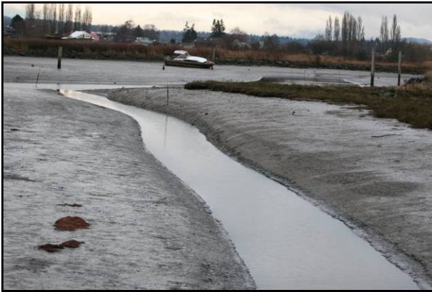
Figure16. Drainage channel outside of work area at confluence with Edison Slough.
