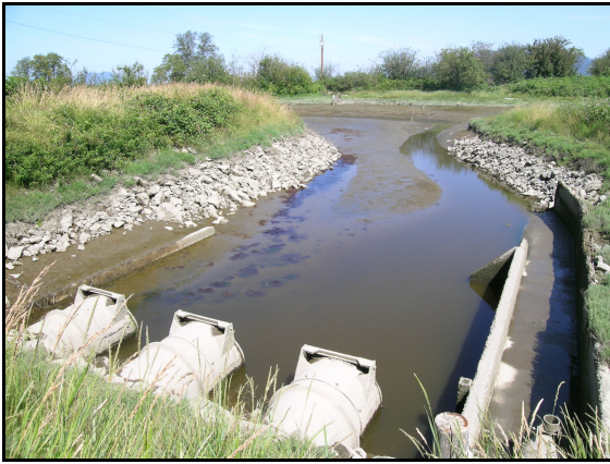
Figure 10. Tidegate Complex 25 side channel to Edison Slough.
