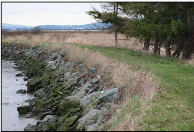
Figure 17. Typical dike bank and site access.
