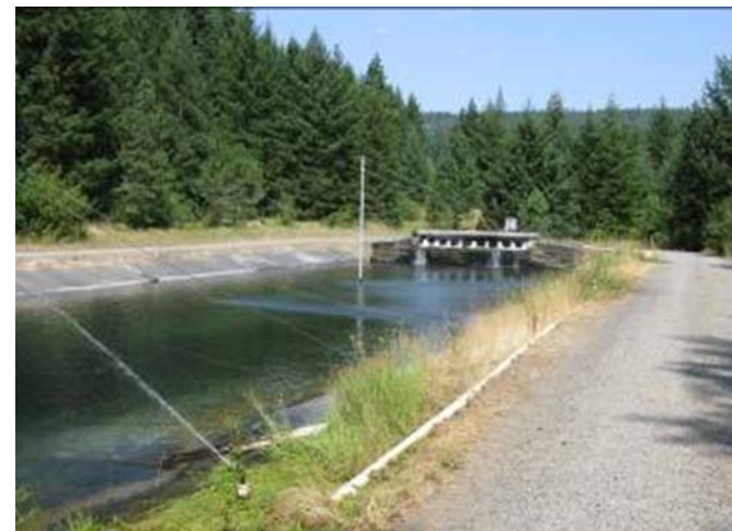
View 7. Klickitat Hatchery Site: Existing raceway within the Klickitat Hatchery Complex looking south.
