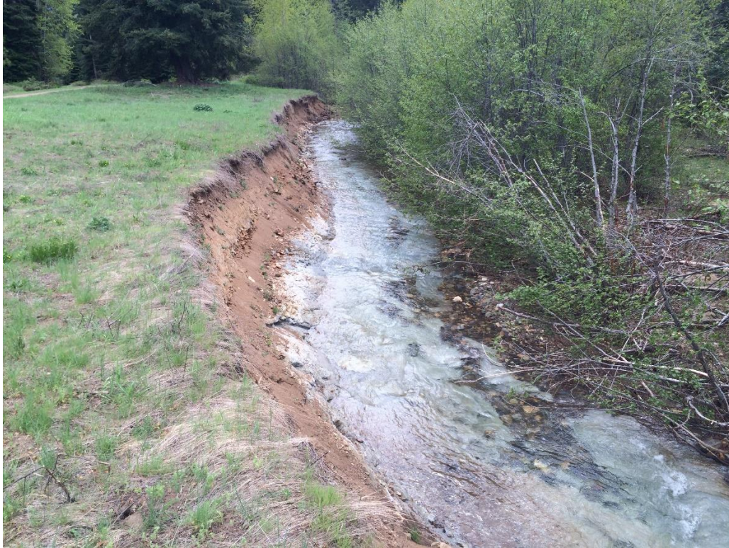
Figure 2. Heavily degraded sub-reach within the Jungle Creek Project Reach. *Note bedrock at streambed surface. Photograph taken May 2016
