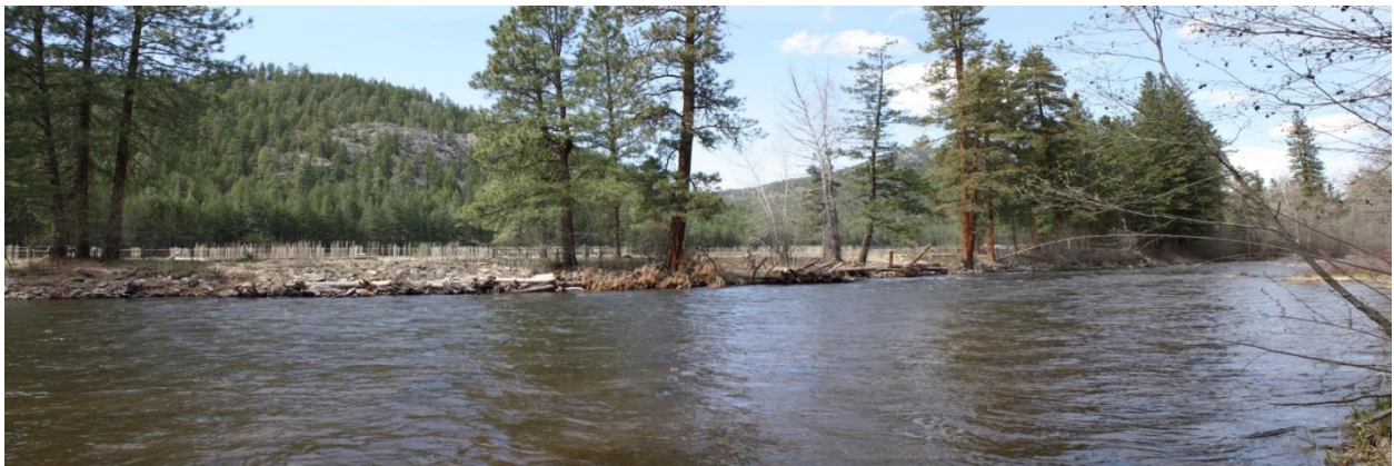
Figure 40. Photograph looking upstream at the constructed log structures on the south end of Eightmile Ranch riverfront.
