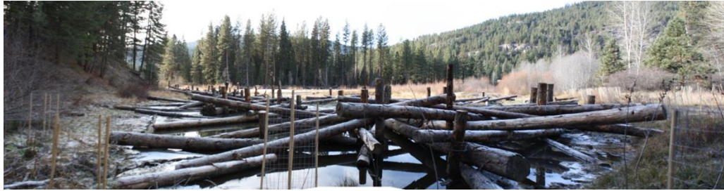
Figure 43: View of Structure 13B from the user-created trail leading to the backwater area.
