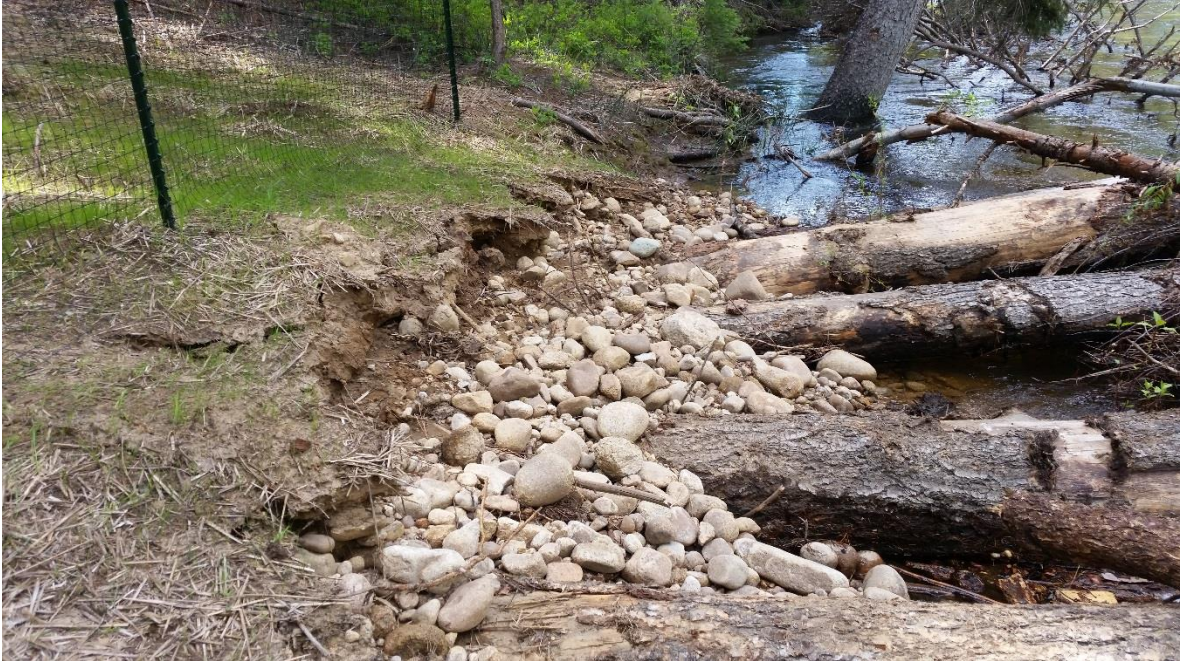
Figure 57: Example of previous in-stream wood placement along the Chewuch River. The bare soil was seeded and the riparian planting were on the other side of the mesh fencing. Rock armoring along the stream bank would help reduce erosion.
