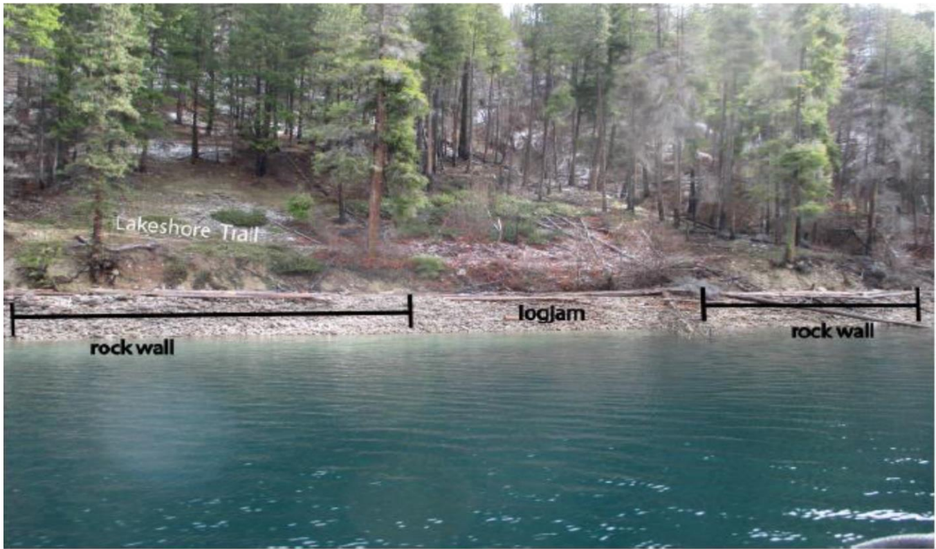
Photo 1. Site 82 during March 2016. Lake Chelan is drawn down about 12 ft, exposing the cobble beach. Note proximity of trail to eroding bank. Proposed solution to protect trail shown.
