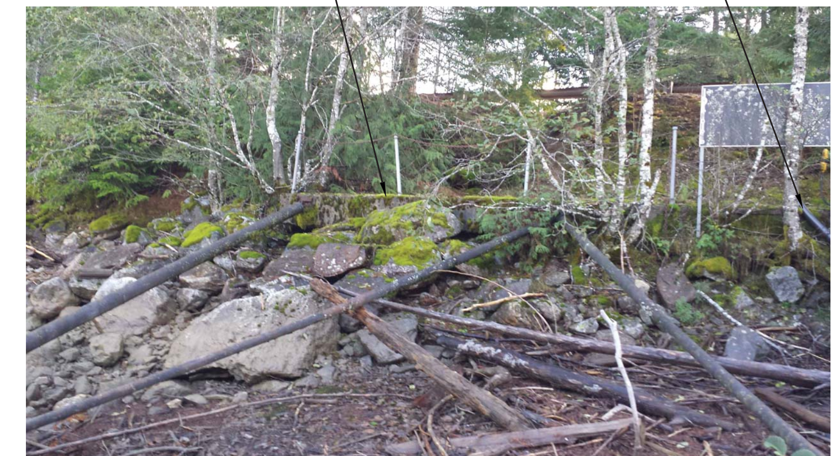
6 C02 | C03 PHOTO #6 - DEMO EXISTING BOATHOUSE ANCHORAGE & APPURTENANCES NO SCALE
