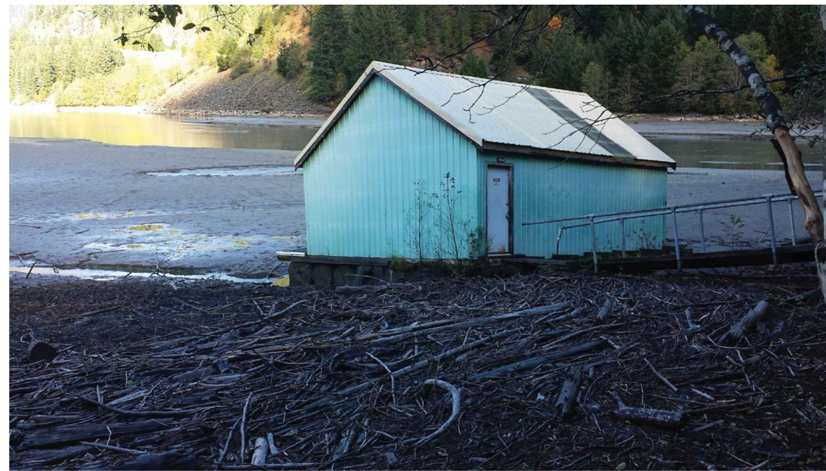
2 C02 | C03 PHOTO #2 - DEMO EXISTING BOATHOUSE & APPURTENANCES NO SCALE
