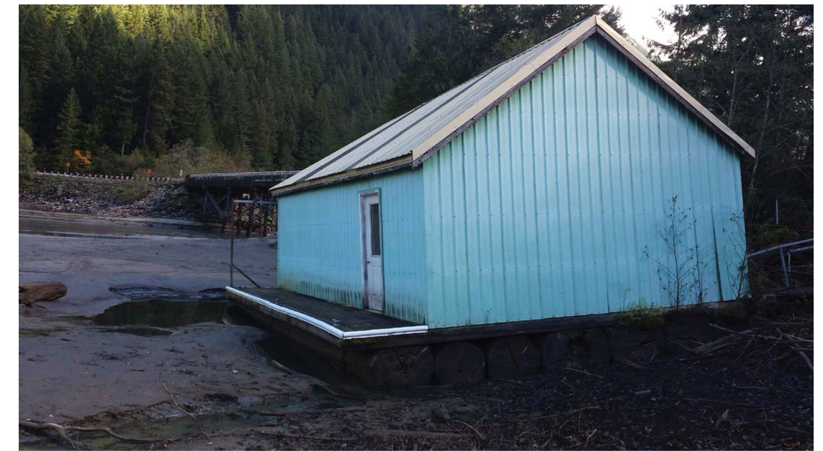
2 C02 | C03 PHOTO #3 - DEMO EXISTING BOATHOUSE & APPURTENANCES NO SCALE
