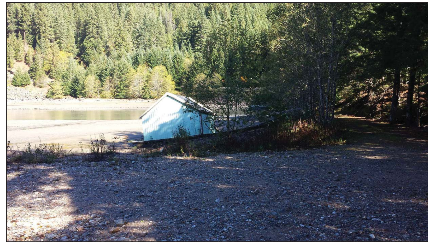
1 C02 | C03 PHOTO #1 - DEMO EXISTING BOATHOUSE & APPURTENANCES NO SCALE
