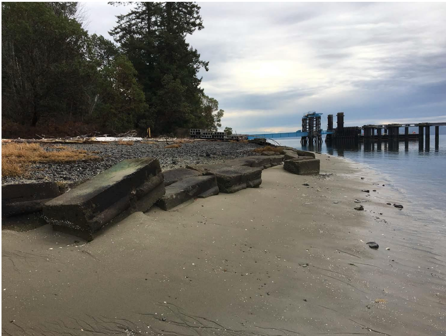
Shoreline debris at Barge Landing
