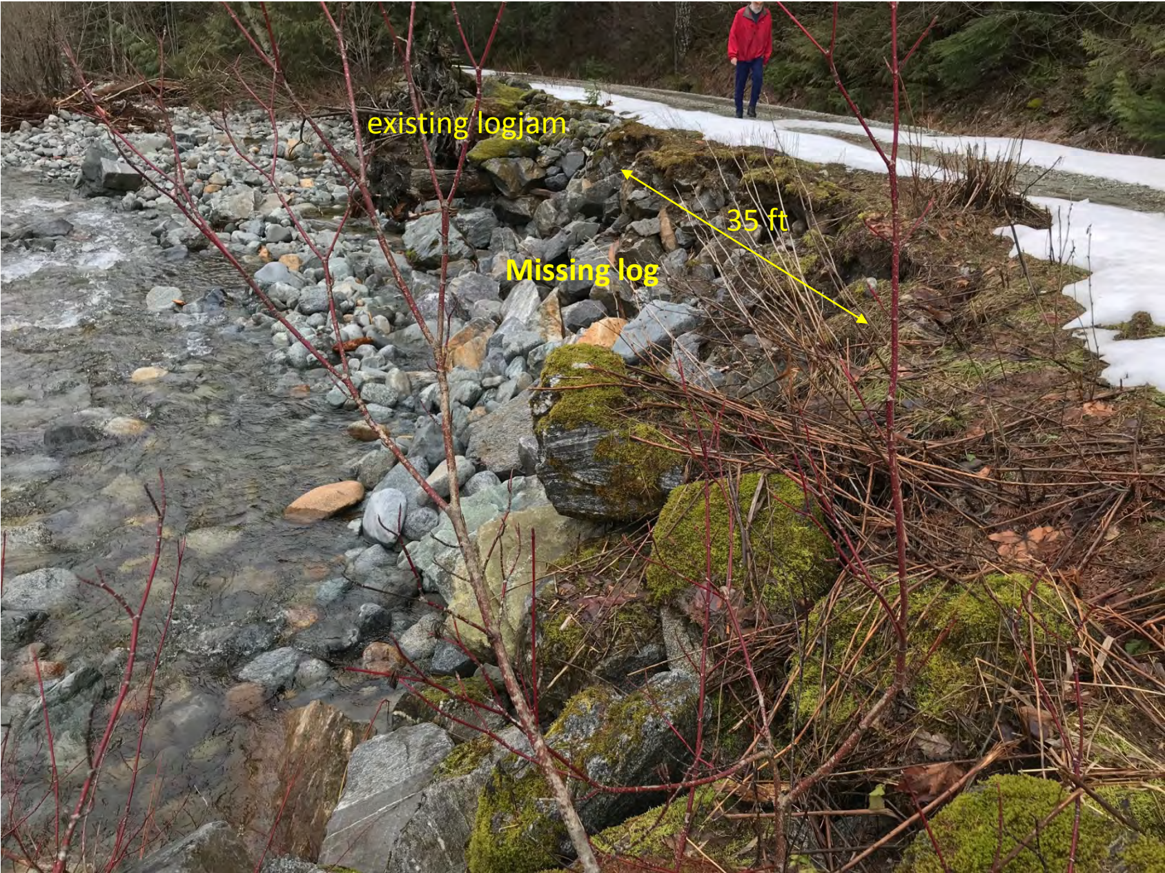
Cascade Road. Site D. View downstream at site of missing log
