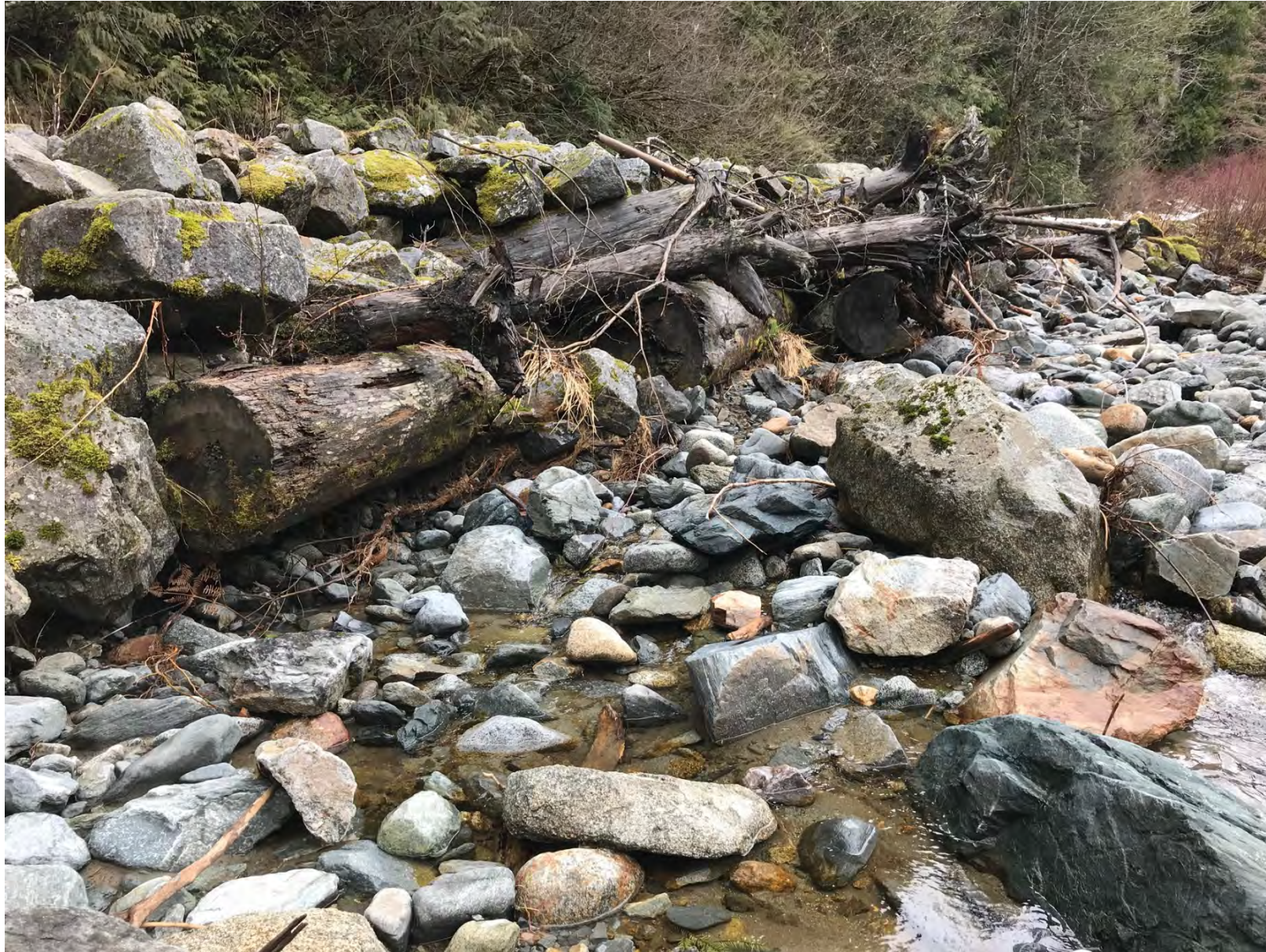
Cascade Road. Site D. View Upstream of Intact Logjam
